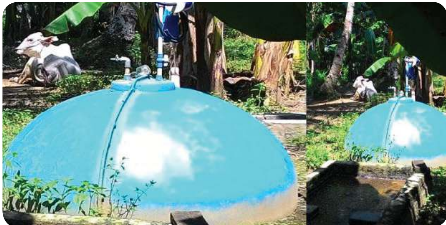
Gambar 2.7 Digester biogas kotoran sapi
