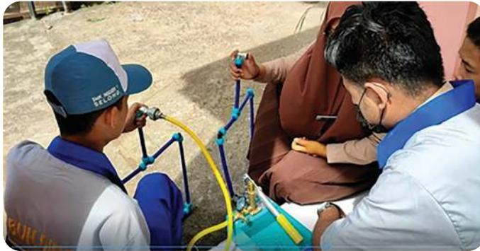
Gambar 3.22 Test Pump Instalasi Pipa PeX
