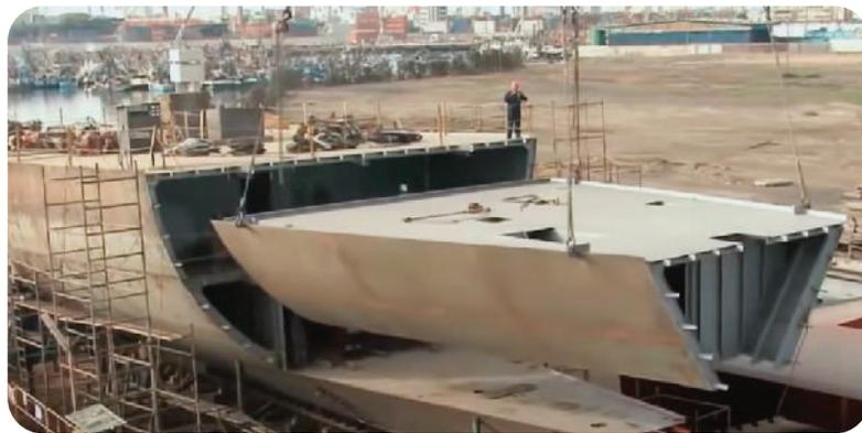
Gambar 2.9 Proses *Erection*
